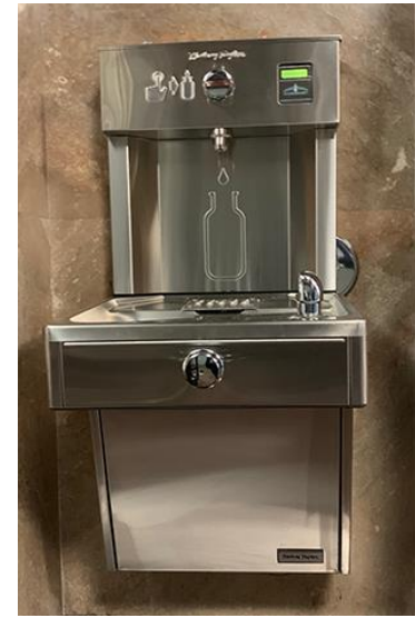
Hydration Stations Installation
