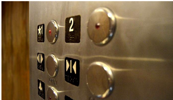
Elevator Condition Assessment and Modernization Plan
