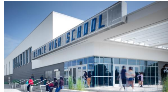
Venice HS Comprehensive Modernization
