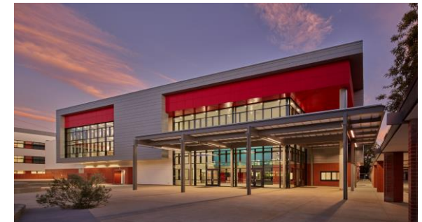
Cleveland HS Comprehensive Modernization
