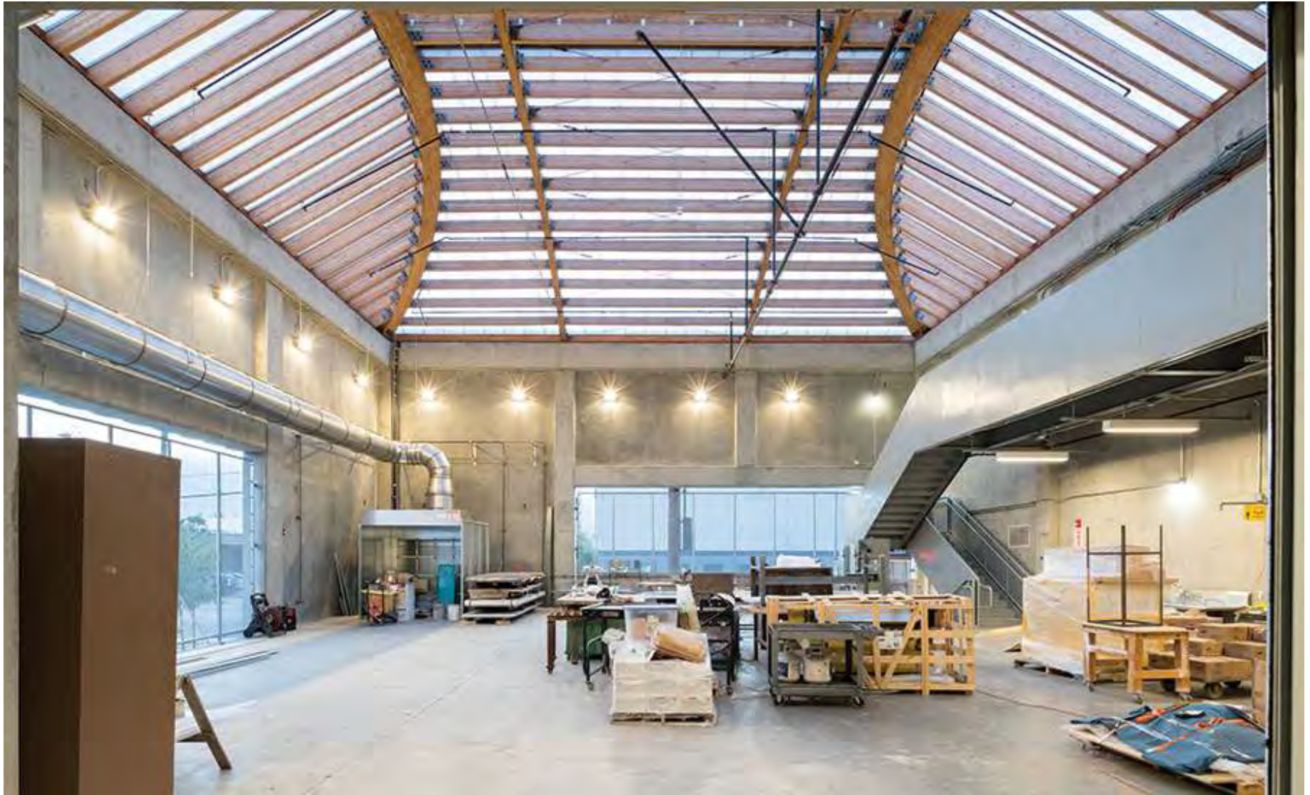
The architecture features an innovative roof and polycarbonate skylight systems.
